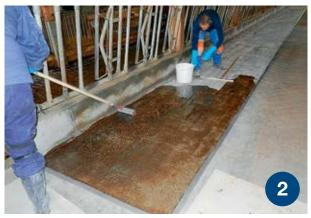
All DeLaval Plast<sup>™</sup> floors and walls are built-up with a primer applied on a dry, clean surface. Easy to apply with roller or squeegee.
