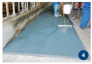
4. The top coating gives the final finish to longlasting surfaces that will remain easy to clean and safe.
