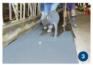
To make a smooth feeding table the primer is followed by a mixture of DeLaval Plast<sup>™</sup> coating and high-quality quartz sand. For walls, two layers of DeLaval Plast<sup>™</sup> colour are rolled on.
